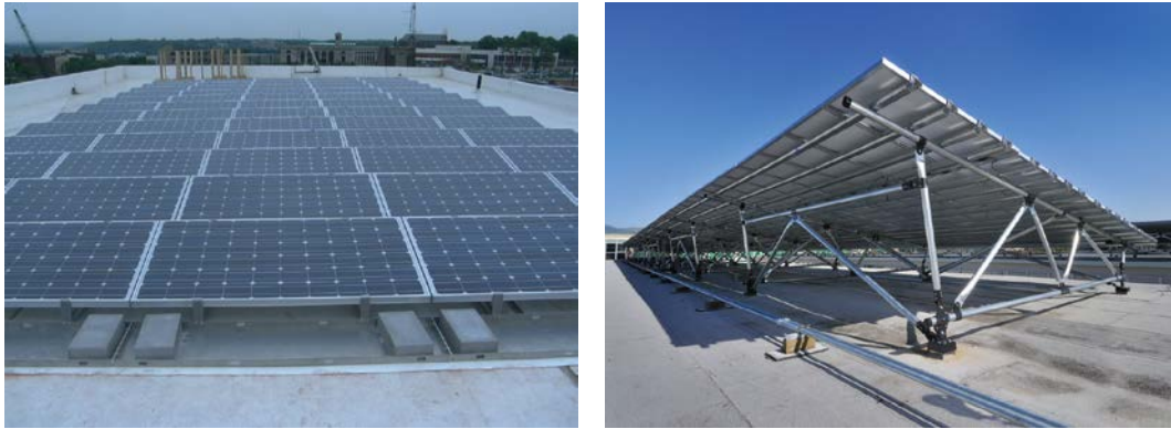
Figure 1.3: A ballasted system (left) on the left with concrete blocks, attached system with metal supports (right).
