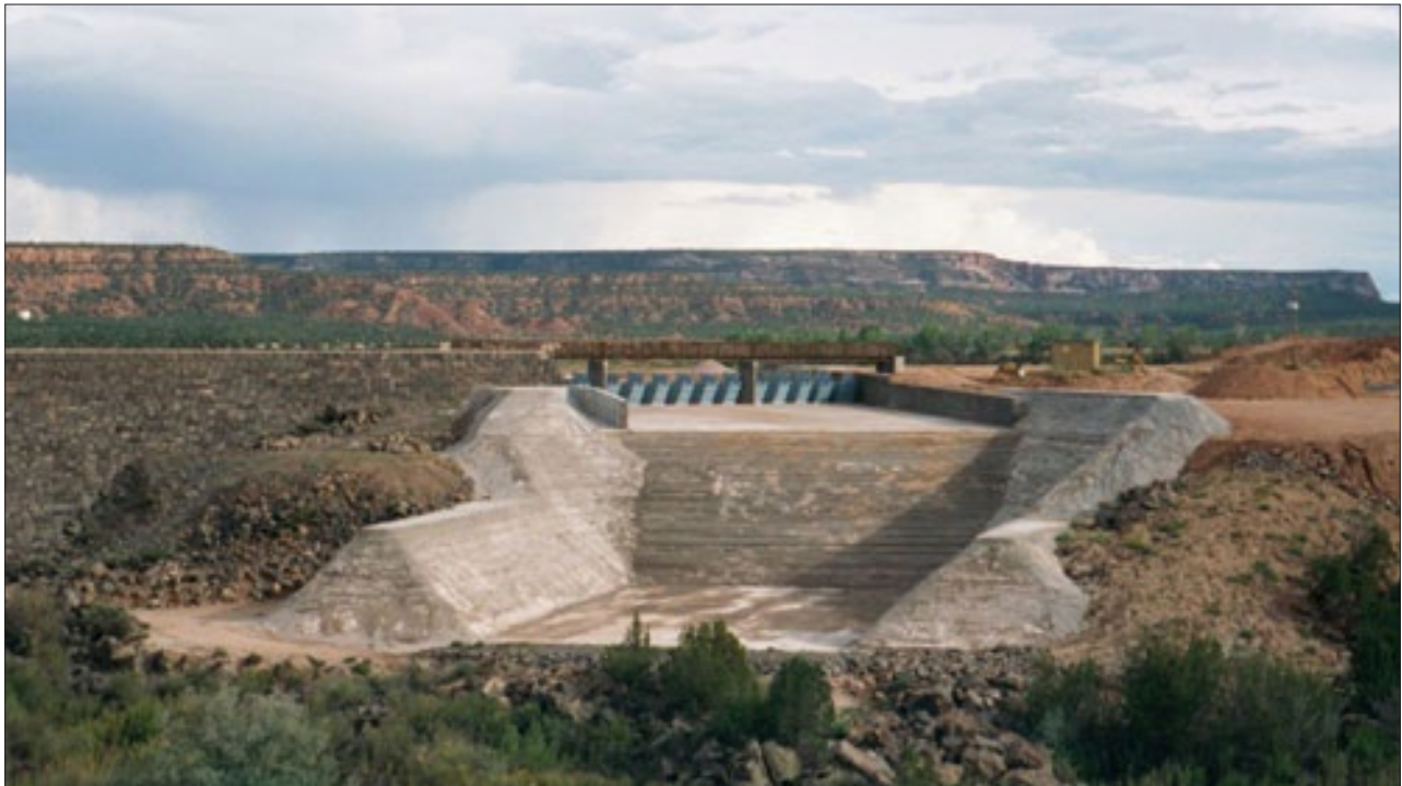
The Black Rock Dam in the Black Rock Irrigation Project. Photo source: Gannett Fleming (2002); reproduced with permission of Gannett Fleming, Inc.
