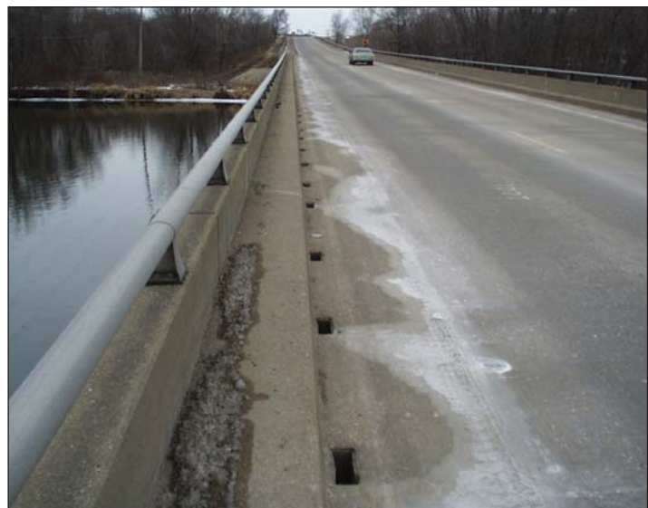
Figure 1. Salt residue left after deicing treatment; note drains and river. Source: Photo used with permission of Chesapeake Stormwater Network.
