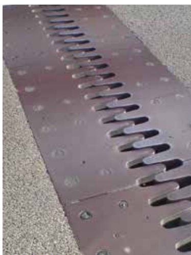
FIGURE 3.10: Bridge expansion joint
